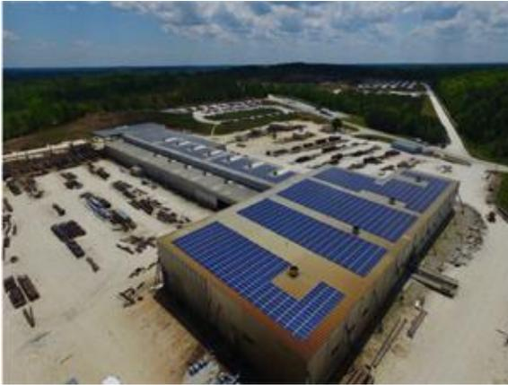
The largest commercial rooftop solar array in the state of Alabama was recently completed. The rooftop system includes 2,296 solar photovoltaic panels providing 746 kW of power to SteelFab's Roanoke, AL steel fabrication plant.
